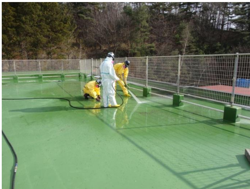
Fig. 20. Manual high-pressure washing of paved areas (source: Miyahara et al., 2012: 15)
