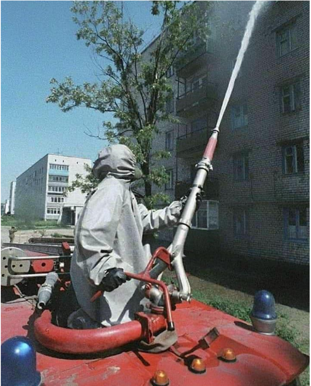
Fig. 5. Washing of buildings in Chernobyl (source: Uatom, 2023)
