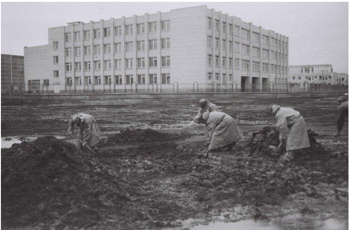
Fig. 4 Manual topsoil removal in Chernobyl (source: Uatom, 2023)
