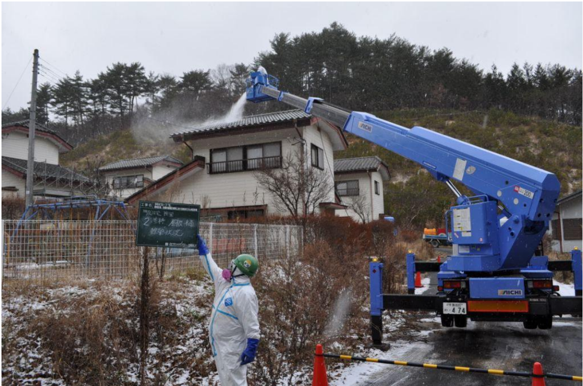
Fig. 21. High-pressure washing of buildings (source: Miyahara et al., 2012: 14)
