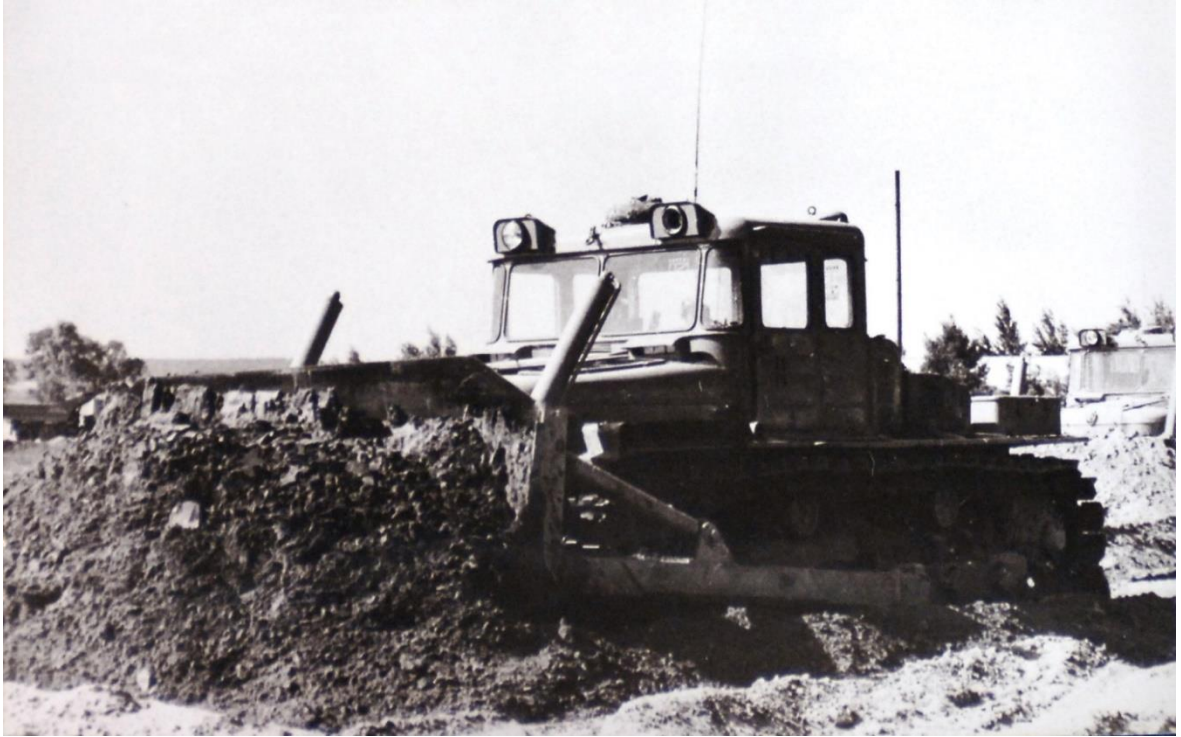
Fig. 3. Topsoil removal using heavy machinery in Chernobyl (source: IAEA, 2011 – Imagebank)
