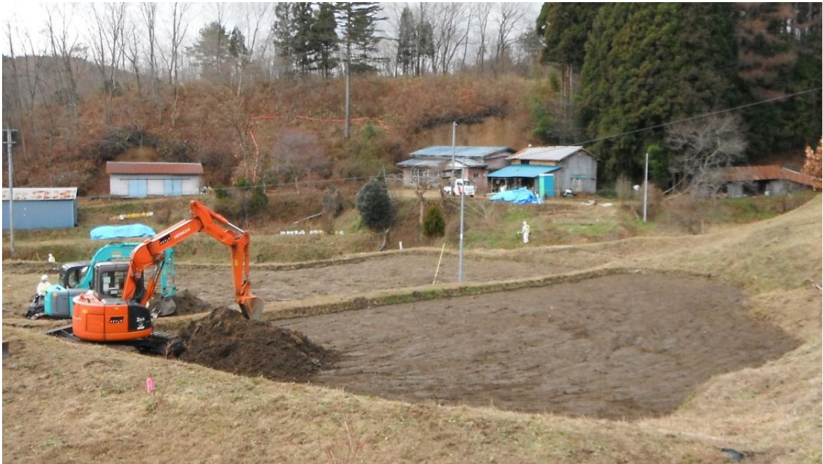
Fig. 16. Topsoil removal (source: Miyahara et al., 2012: 13)
