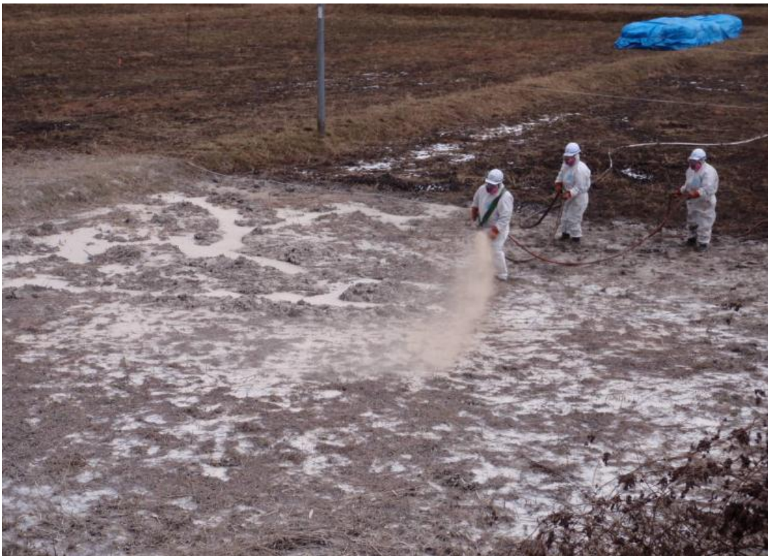
Fig. 15. Soil solidification (source: Miyahara et al., 2012: 13)
